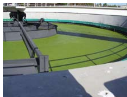
This water treatment plant uses the base sodium hydroxide, NaOH, to remove impurities from the water.
